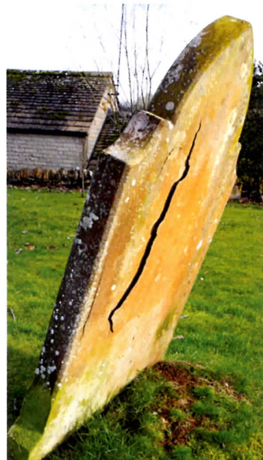
Fig.4: Frost splitting of gravestone, Naunton churchyard.
