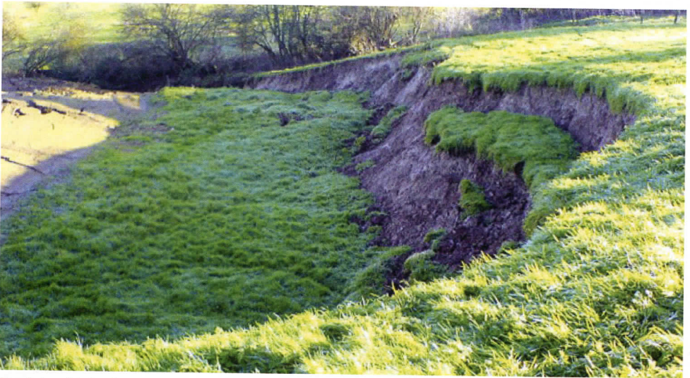
Fig. 4: Landslide above the Windrush valley (Dec. 2006), south of Bourton on the Water. Height of the arcuate head scar ~3m. For location see Figs. 5,6.
