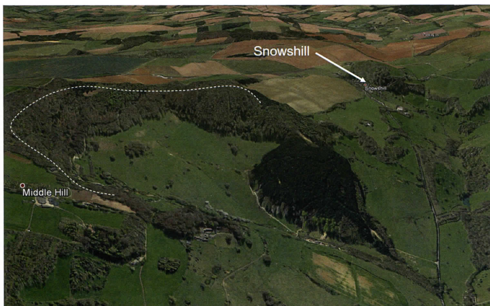
Fig. 3: Google Earth view of a possible landslide on the east side of the valley between Broadway and Snowhill, looking South. The white dashed line highlights the arcuate scarp or slip face, whilst Dulverton Wood (the forested hump in the middle of the slope) could be a block of oolitic limestone detached from the crest of the scarp. The slip face is ~1 km in diameter.
