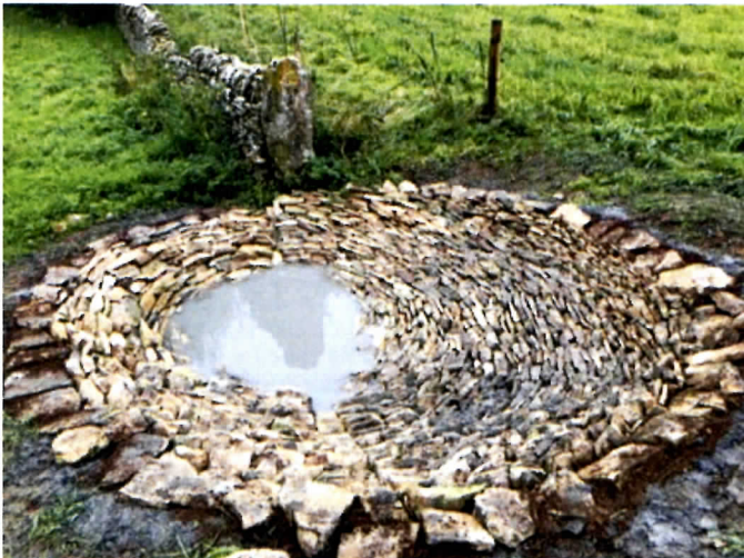
Fig. 4: Reconstructed Dew Pond, showing the stone lining to protect the clay seal below from puncture by sheep/ cattle hoofs. Photo from farmoffice@firfarm.co.uk
